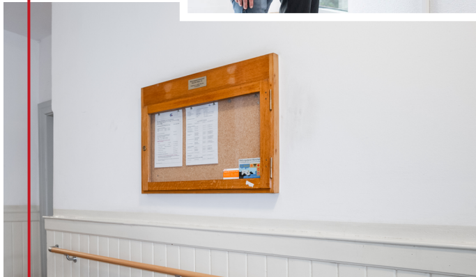
Before the conversion a wooden sign hung in the hallway
