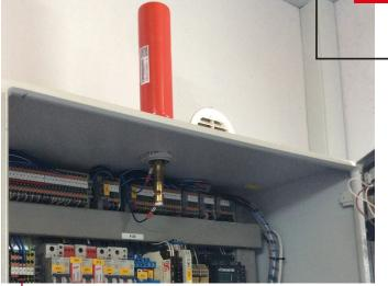
In order to ensure the operational safety of their electrical systems, the electrical engineering and preventive fire protection teams sought advice from Multicomsystem OHG in Hilden. The focus was on fast, and residue-free, fighting of any fires in their electrical systems. Their system includes control cabinets, control devices and pump systems. The aim being to keep any fire damage to a
