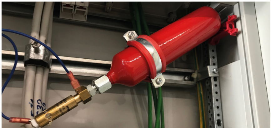
Remote controllable AMFE at FTI Group
