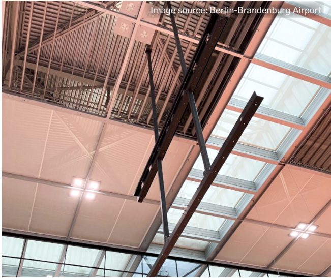
The metal substructure on which the LED cabinets could be installed.
