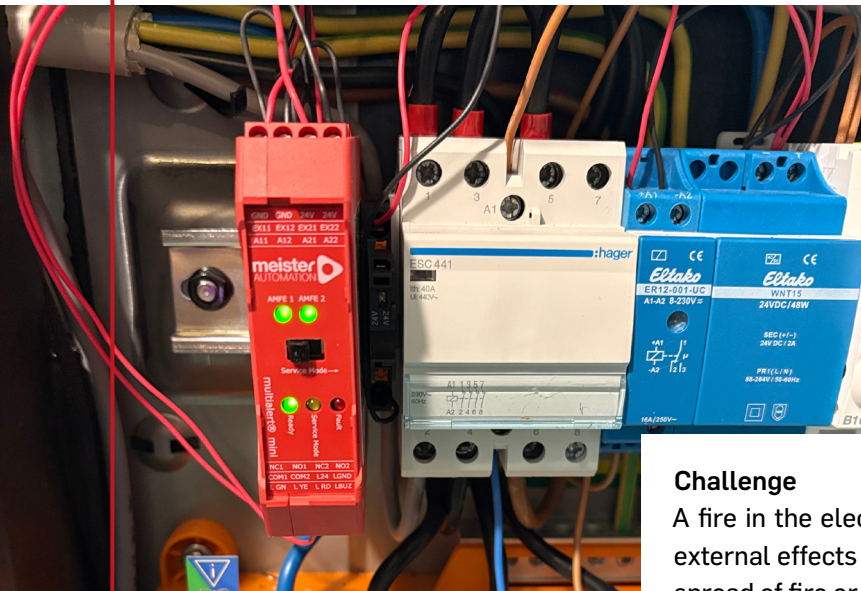
Shutdown function of the electrical cabinet (including for the heat pump and electric auxiliary heating) as well as disabling the activation of the emergency power supply from the storage battery.
